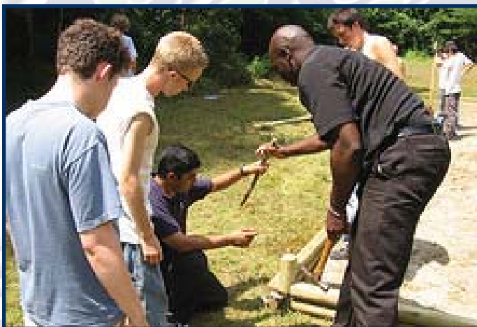
MSU scholars construct a sand volleyball court during Community Service Day.
